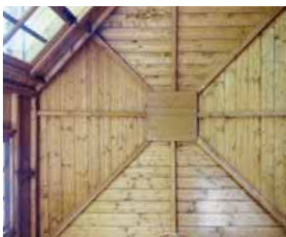
Internal roof structure
